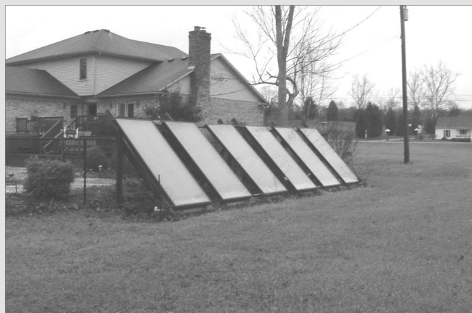
Figure 10.2: Six flat plate solar collector panels are located to the south of this swimming pool. The solar collectors are hidden behind a screen so that they cannot be seen from the pool itself, Andy McDonald (right photo)
