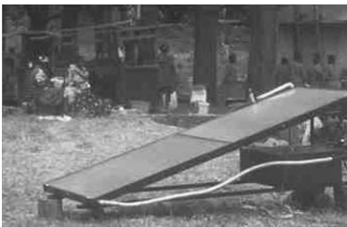
Figure 12.15: Solar water pasteurizer Safe Water Systems
