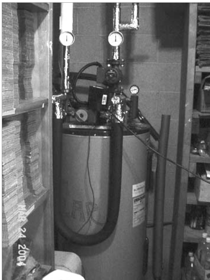
Figure 7.6: A conventional electric water heater tank uses an external heat exchanger in the solar water heating system at the ASPI office in Mt. Vernon, Kentucky, Andy McDonald
