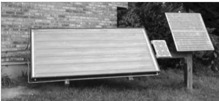
Figure 8.6: This flat plate solar collector (left) is mounted on the ground outside a home in northern Kentucky. This glycol antifreeze system uses a small PV panel (center) to pump the antifreeze through the system, John Robbins
