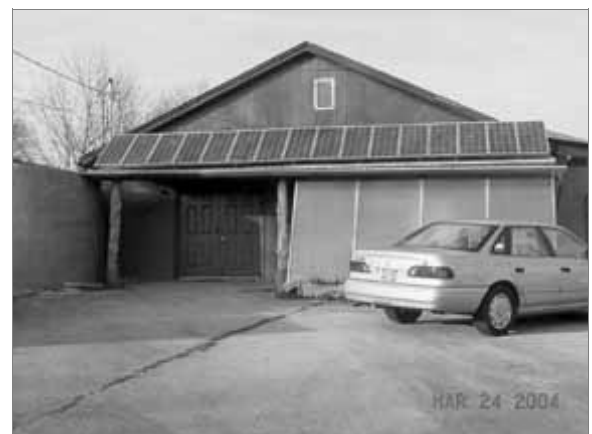
Figure 3.10: This grid-intertied PV array at the office of Appalachia- Science in the Public Interest in Mt. Vernon Kentucky was one of the first net-metered systems in the state. The inverter is shown at left and the PV array above the entrance at right, Andy McDonald
