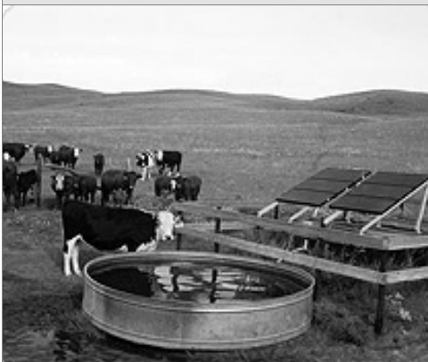
Figure 3.6: PV-powered water pumps provide water for livestock.
