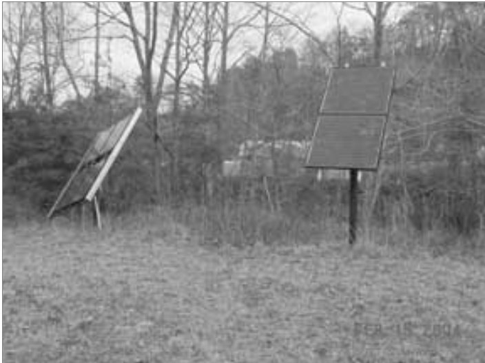
Figure 5.3: The tracking PV array on the left is facing the afternoon sun, while the fixed array on the right faces due south, Andy McDonald
