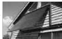
Figure 7.5: Evacuated tube collector doubles as an awning. Thermomax, Inc.
